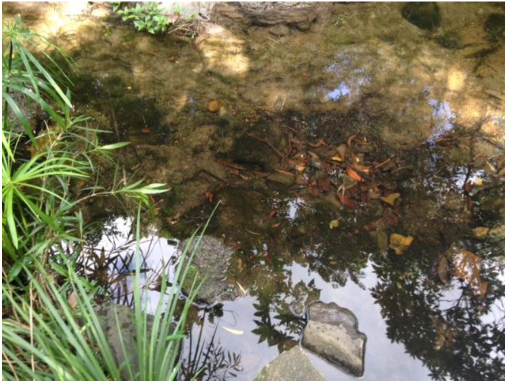
Below Stormwater Culvert
