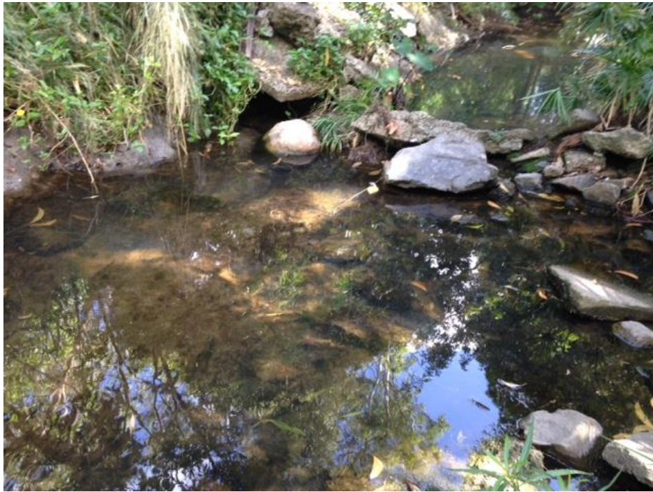
Below Stormwater Culvert
